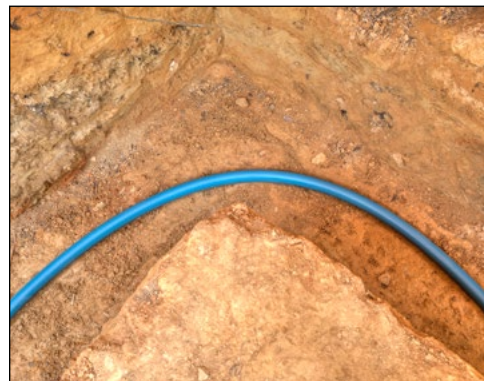
Figure 10.15 PEX Water Service Tubing in Trench
